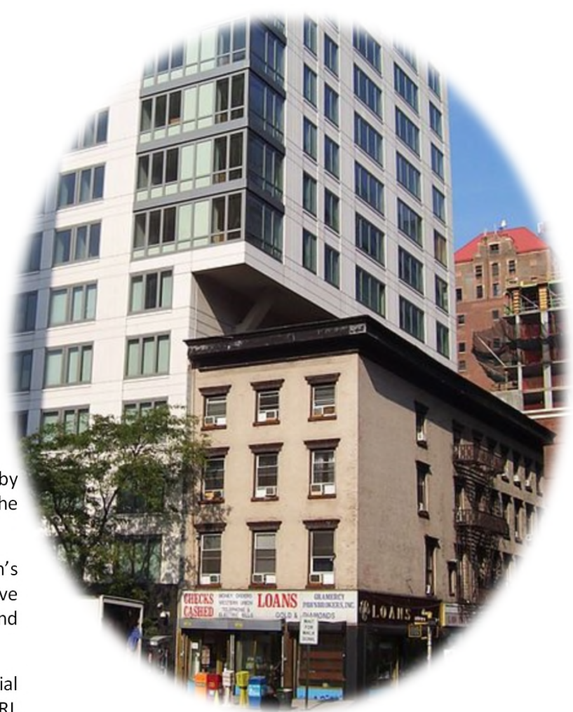
An example of air rights in use: a high-rise building extends over a four-story building.
